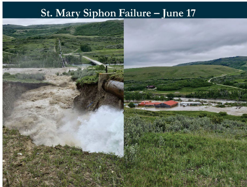
Figure 3-18. Example of a 2024 St. Mary Canal System Failure (MRJBOC 2024)
