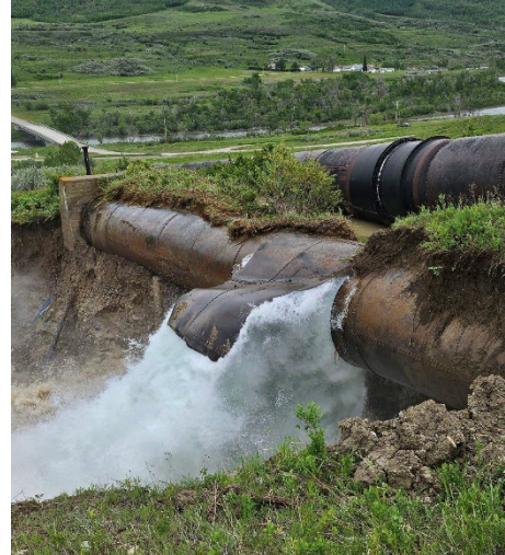
Photo 1. Failure of St. Mary Siphon
