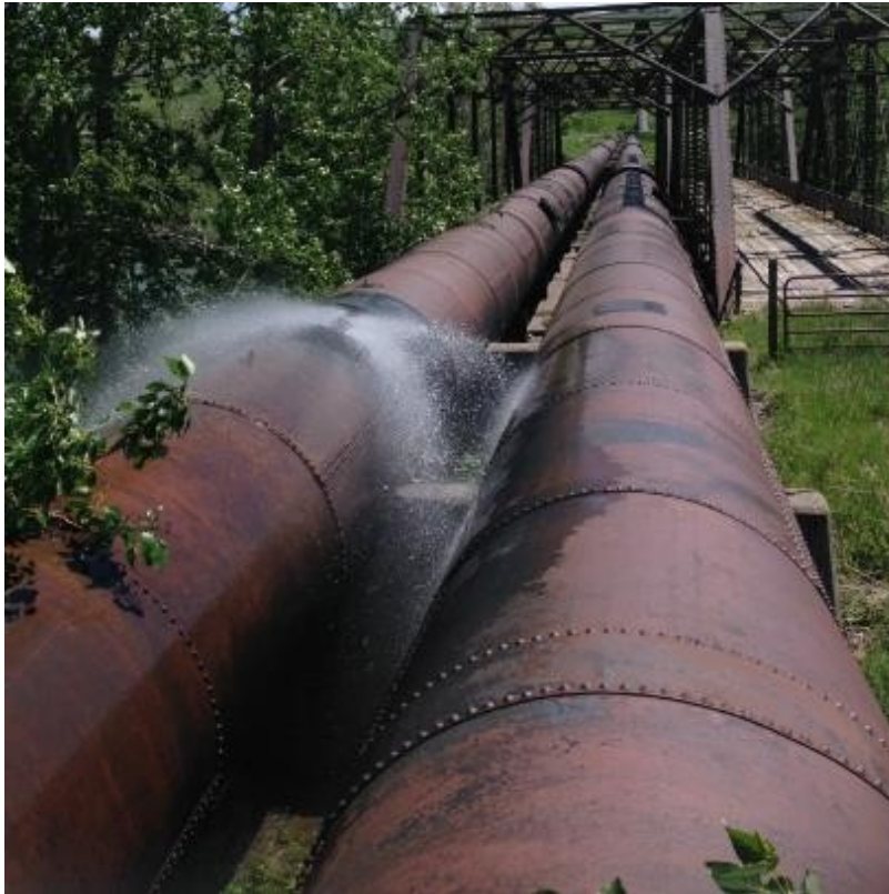
Figure D3-4. St. Mary Siphon Leaking Steel Barrels
