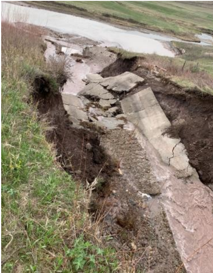
Figure D3-16. Drop Structure 5 Failure 6
