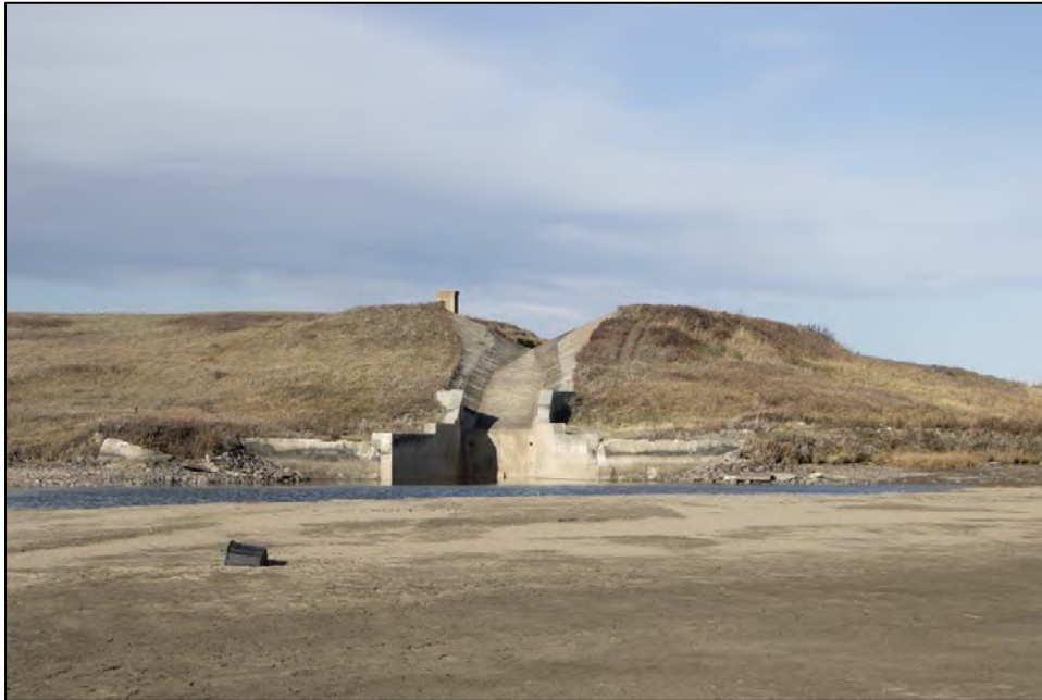
Figure D4-17. Site 24GL155 Drop Structure 1
