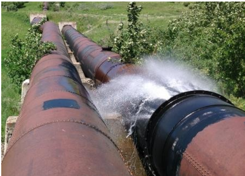
Figure D3-4. St. Mary Siphon Leaking Steel Barrels
