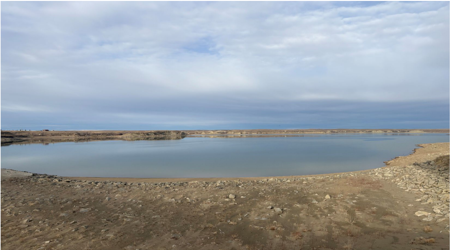
Fresno Dam, March 2026
