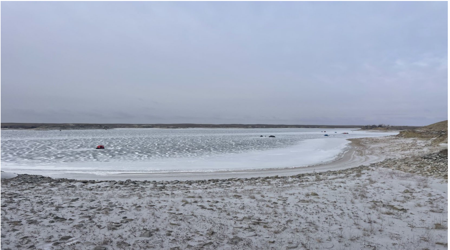
Fresno Dam, January 2026
