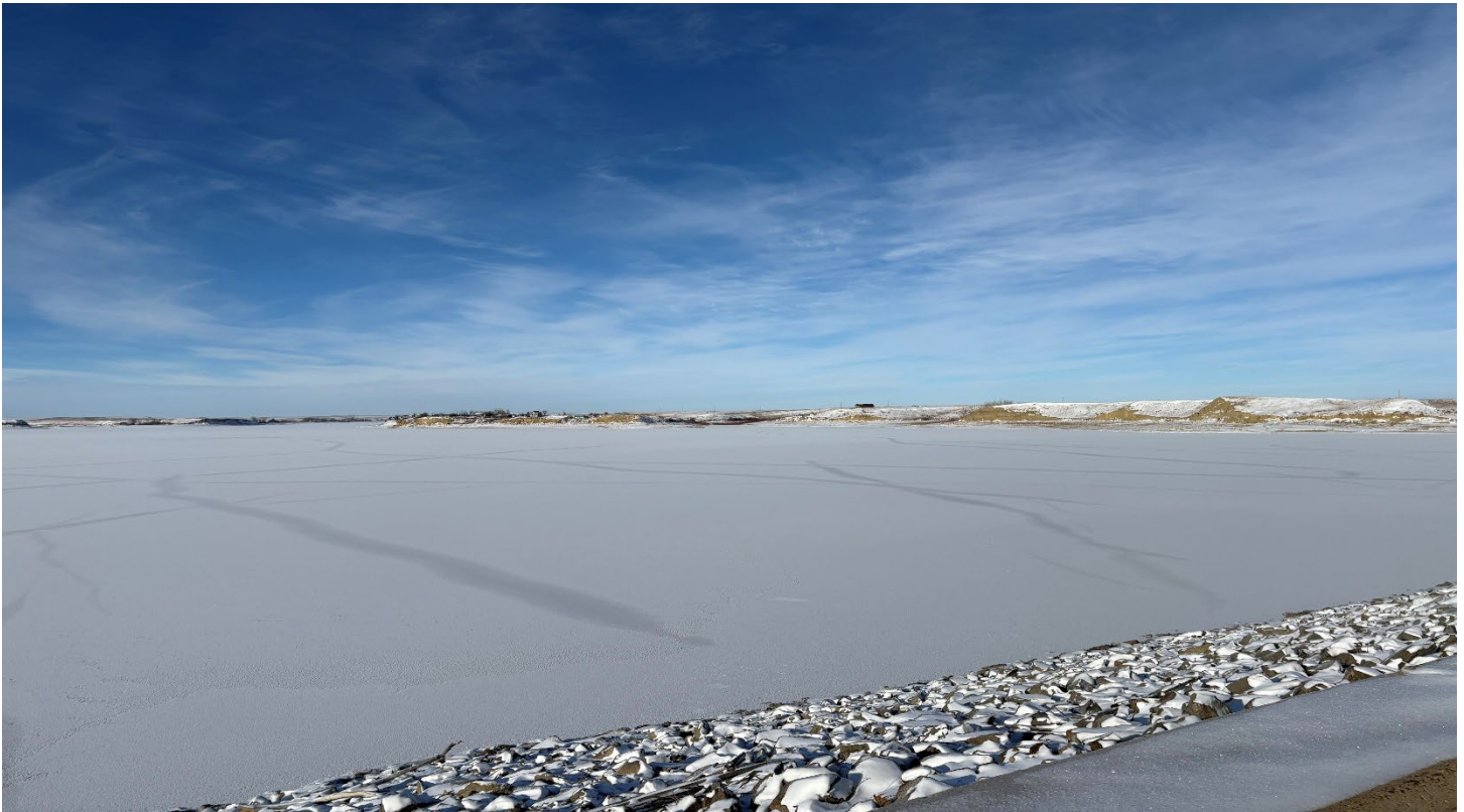
Fresno Dam, January 2026
