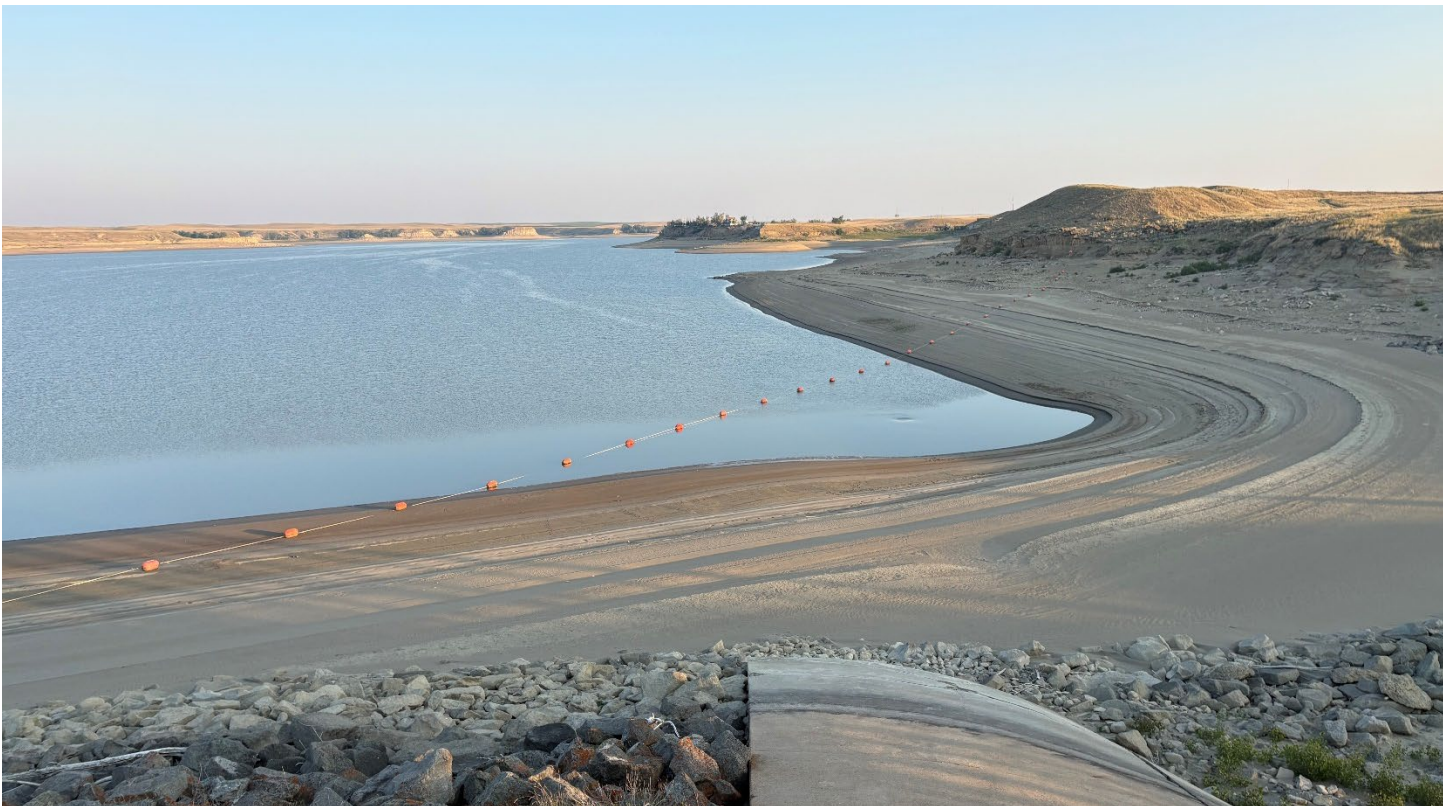
Fresno Reservoir, June 2025
