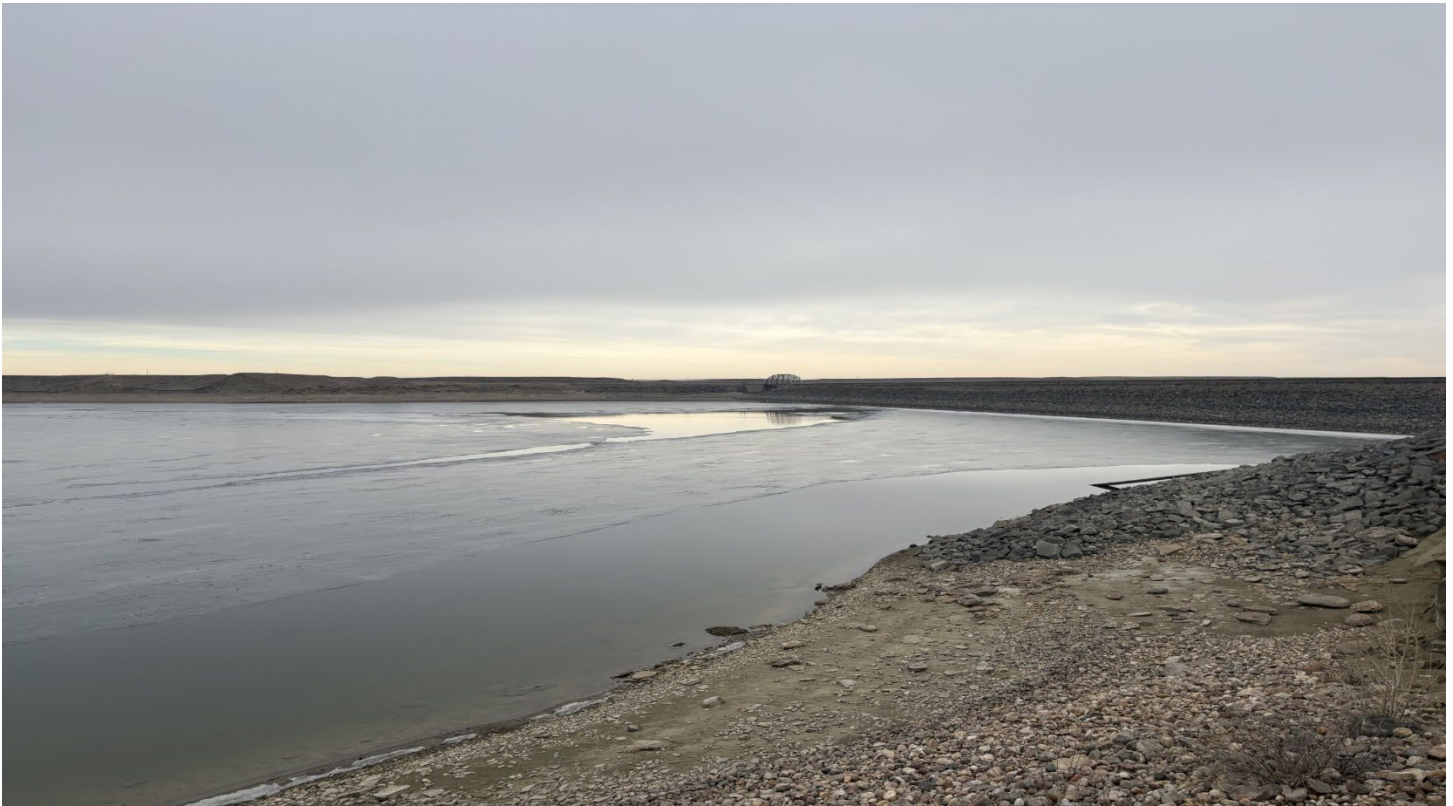
Fresno Dam, March 2026
