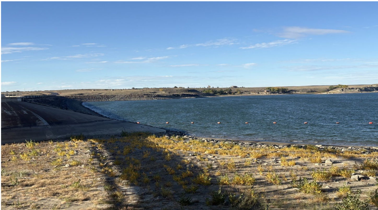
Fresno Reservoir, October 2025
