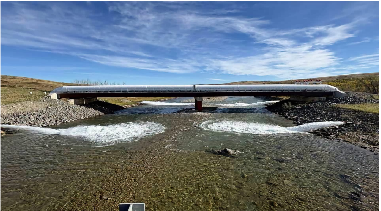
St. Mary Canal Siphons, September 2026
